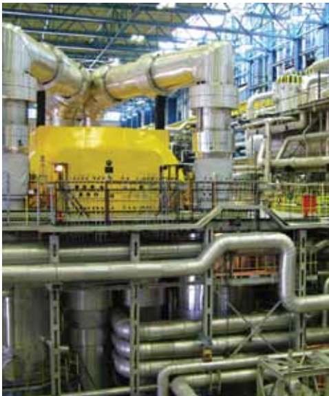
Images courtesy of Paks Nuclear Power Plant
